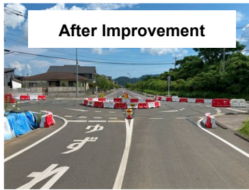
■ Entry Point A
